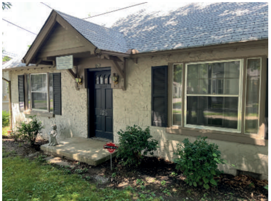
The first building for New Day Christian Distributors
